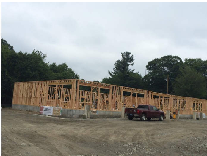
Photos taken in July of the construction going on at Long Hill Marketplace, where Mex on Main will be located.
